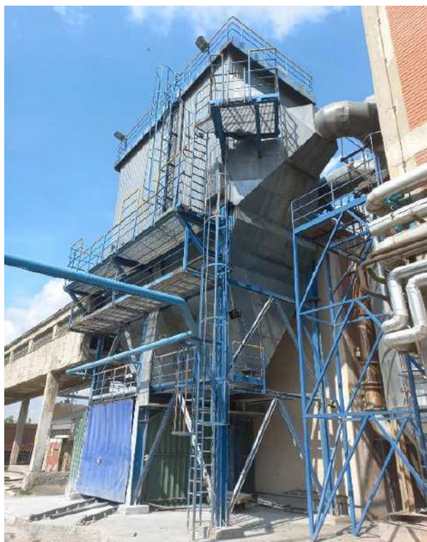
Figure 1. Facility and electrostatic filter where ash is collected, Dijamant Zrenjanin
